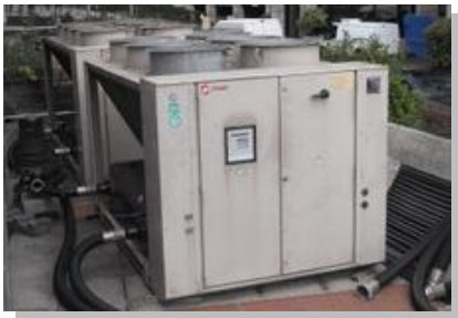
Trane emergency chiller hire system, serving building air conditioning and computer rooms
