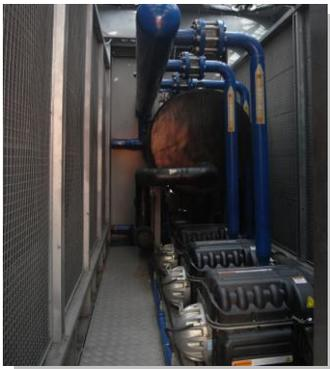
Internal view of the rental unit showing the compressors and flooded evaporator
