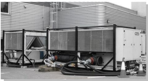
The modified Modular SRAT chiller installed providing emergency process cooling
