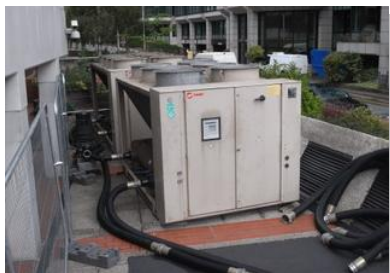
The completed installation
