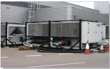
The completed installation
