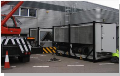
Chiller sections being installed
