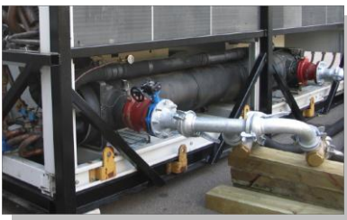
The main module including the evaporator and water connections
